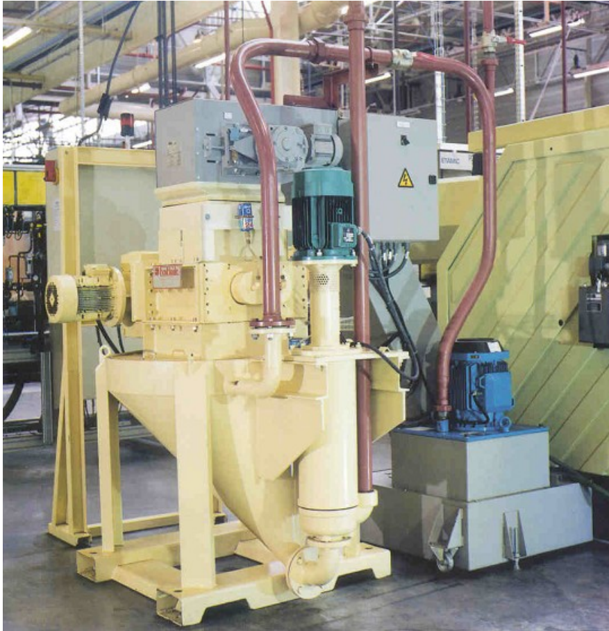
Recovery station with crusher (ERNAULT machine tools at STA)
